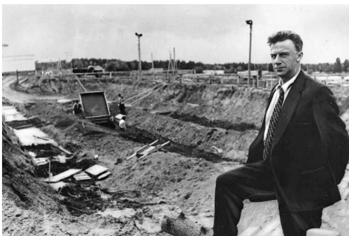
S. Sobolev, the construction site of the Mathematical Institute in the Novosibirsk Akademgorodok.
